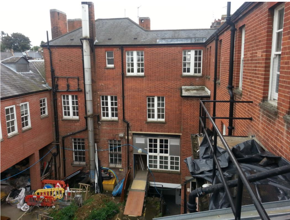
Image 4 View of rear elevation
